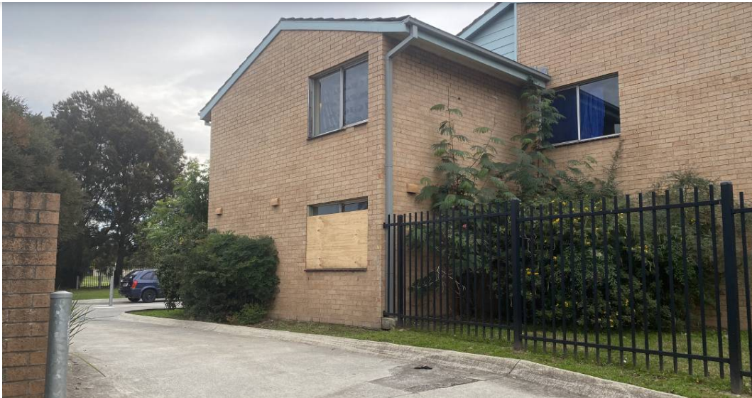
📷 The bedroom window boarded up at 21 Kully Way.
